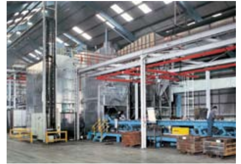
CT-6 blast cleaning machine with noise abatement cabin and sorting belt
